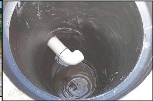
Looking down into the collection basin where tile output is collected in a bucket for nitrate analysis.
